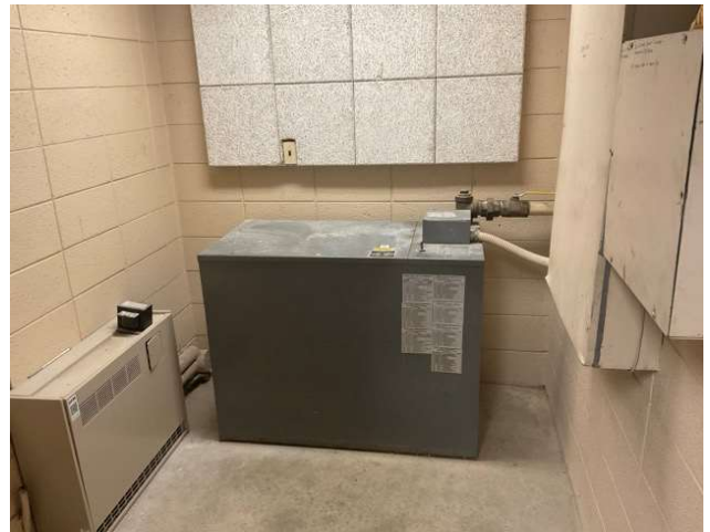
22 - ELEVATOR MACHINE ROOM
