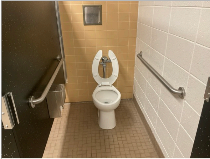
TOILET STALL OVERVIEW
