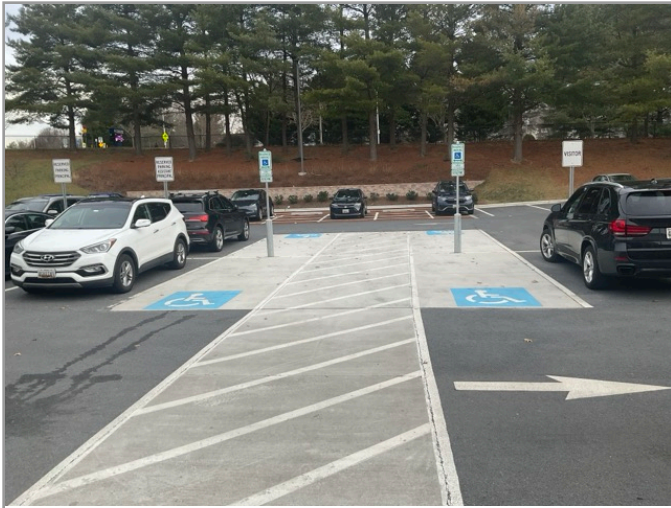
OVERVIEW OF ACCESSIBLE PARKING AREA
