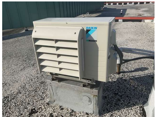
30 - SPLIT SYSTEM DUCTLESS
