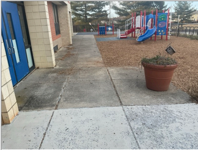
ACCESSIBLE ROUTE TO PLAYGROUND
